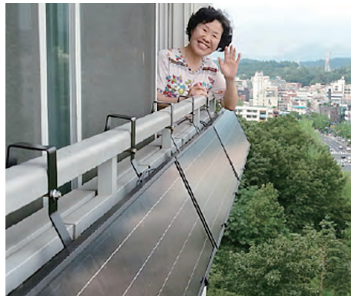
Figure 1: Mini PV System for Apartment block Source: SMG 2015a
